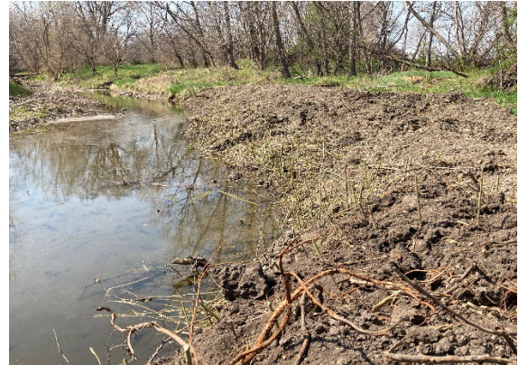
Willow cuttings planted along bank.
