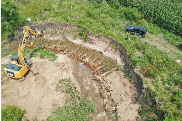
Bank stabilization using rootwads.
