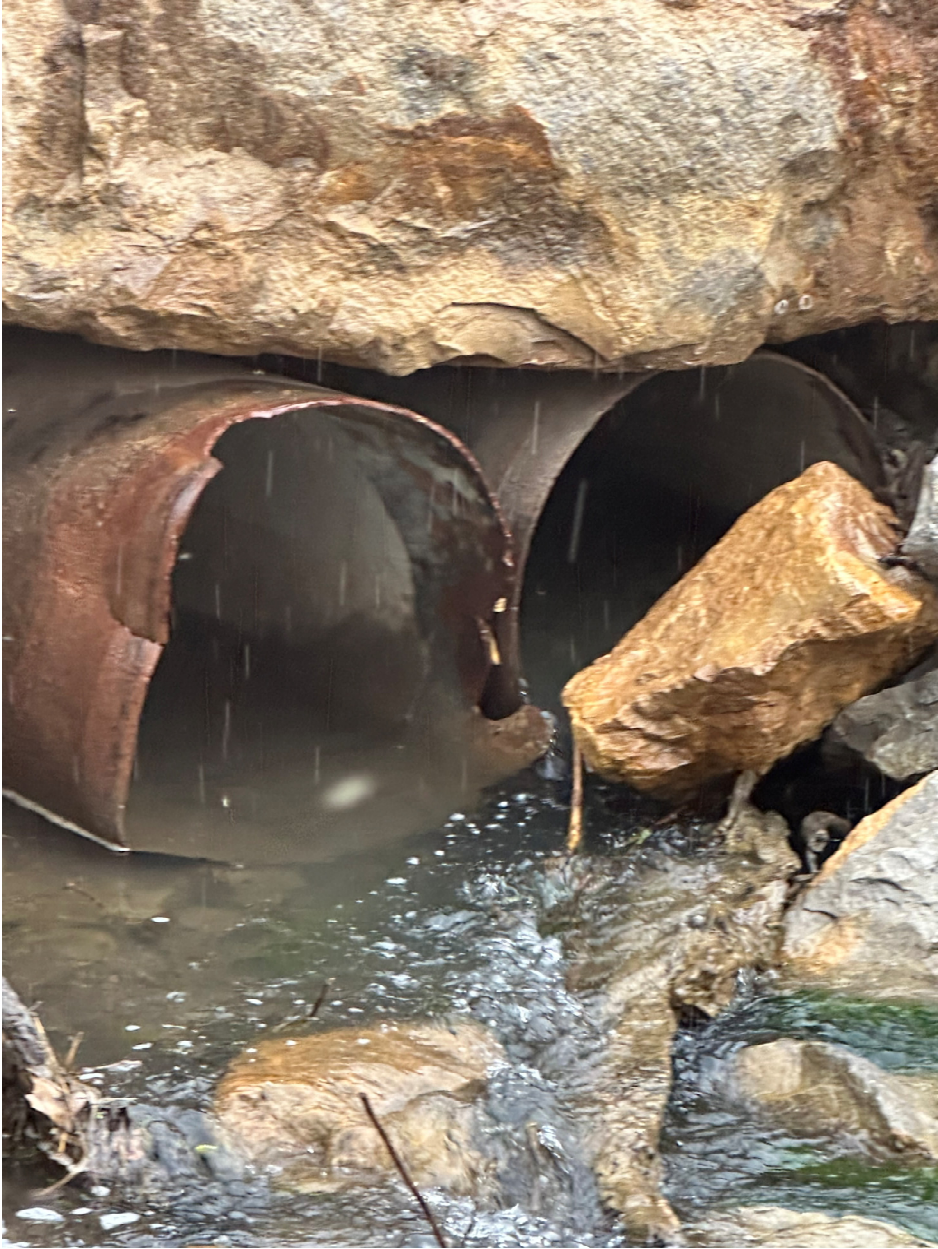
Two 24inch pipes
