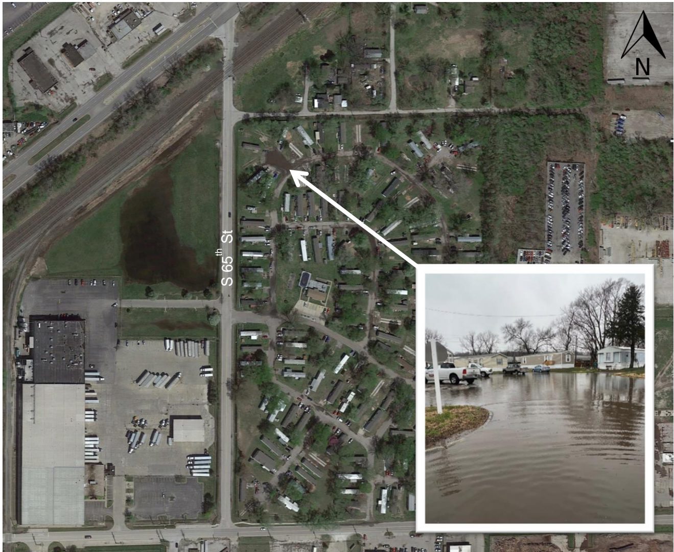
FIGURE 6 - EXISTING CONDITIONS FLOOD PICTURES
