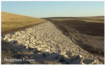
Riprap is a common cover material for embankment dams. This rock cover prevents erosion of dams' upstream faces and may protect during dam overtopping.
