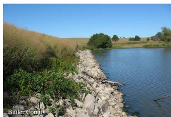
Larger rocks have to be big enough to break the maximum anticipated wave action and also hold the smaller stones. If too small, the rocks will be washed away by waves. If insufficient, the filter material will wash out causing the embankment to erode.
