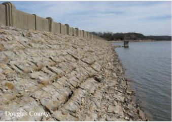
For optimum endurance, use dense riprap stone. In Kansas, limestone and hard sandstone are acceptable for riprap. But most sandstone and shale found in Kansas do not provide the long-term protection needed on dams.
