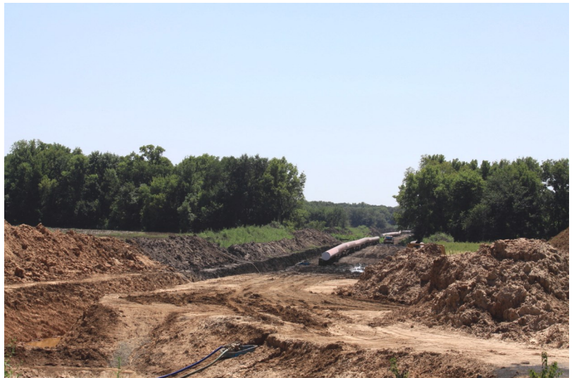
Pipeline work in the floodplain
