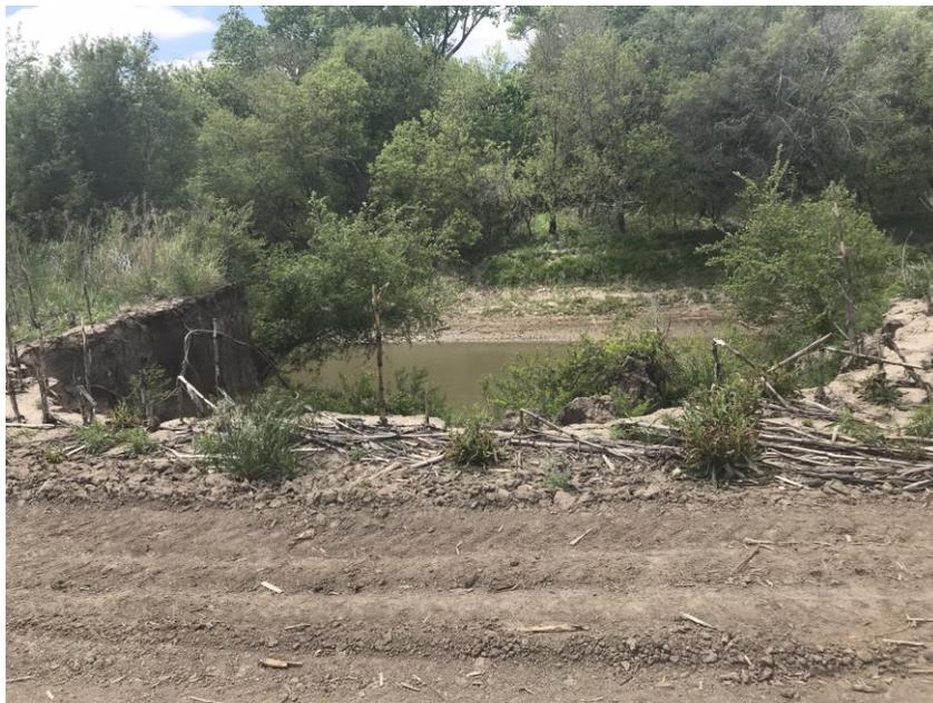
Figure 8. Bank Slumping on Site 22 (Reach 4) in Region of Woody Revetment Installation, May 2020.
